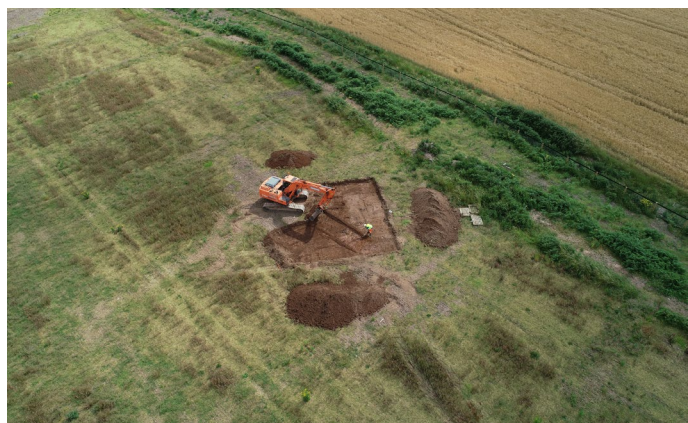
Stripping of topsoil underway at Ballinrea
